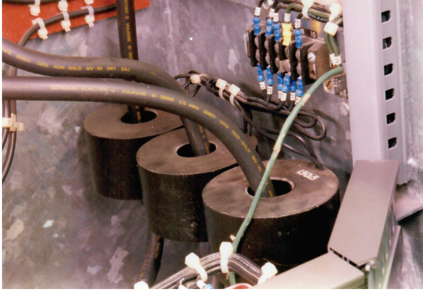
FIGURE 34-10 Current transformers are used to reduce the current to overload heaters.
