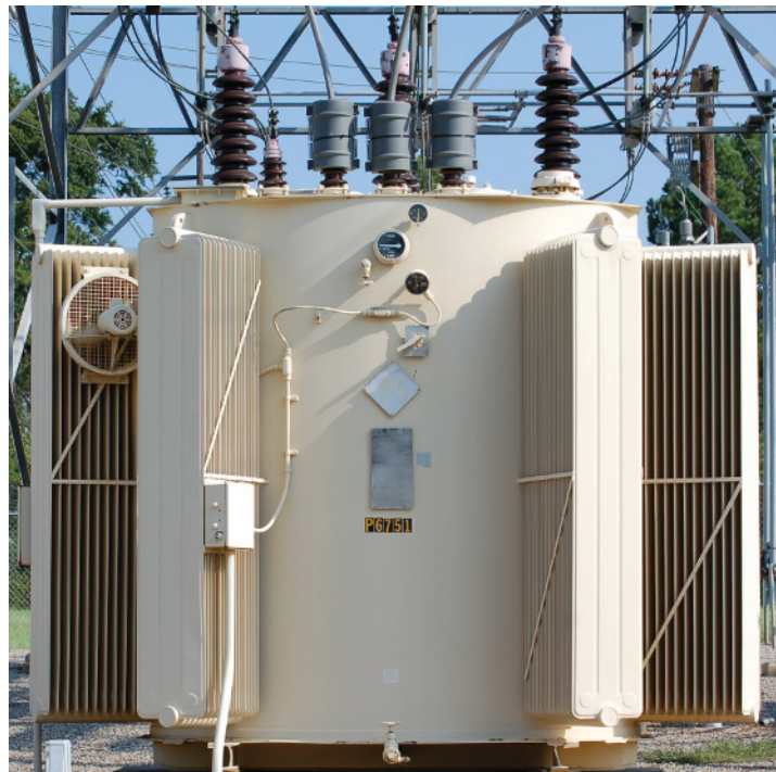
FIGURE 27-43 Three-phase autotransformer.
