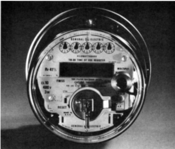
Figure 10-17. Demand Meter with Cover Removed.
