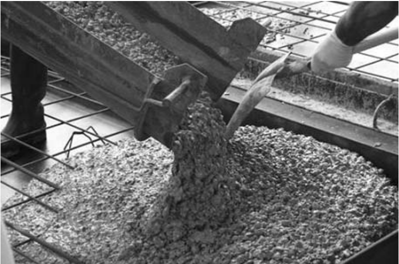
Figure A.13 Application of ready-mix IPC low-strength (25 MPa) and high-strength (+80 MPa) materials developed by Siloxo Pty Ltd (Australia) in conjunction with industry partners.
